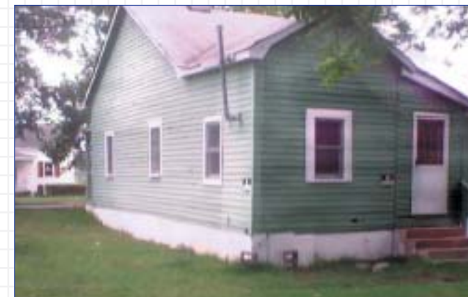
This abandoned home in Wilmington's historic district was gutted and restored to meet Energy Star™ standards.
