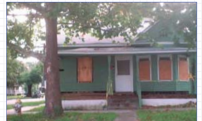
Icynene®, a high-performance insulation, was selected to address the homeowner's strong allergic sensitivity and reaction to mold and mildew.
