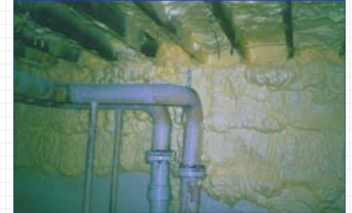
The gaps/cracks were sealed with Icynene® to prevent air leakage and from the above grade exterior.
