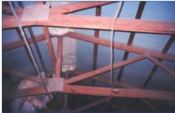
Sealing of the ridge vent with Icynene® Insulation to prevent air leakage.
